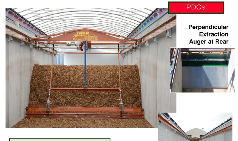
Garage Pellet Storage Bin with Rake & Auger Feed to Boiler
