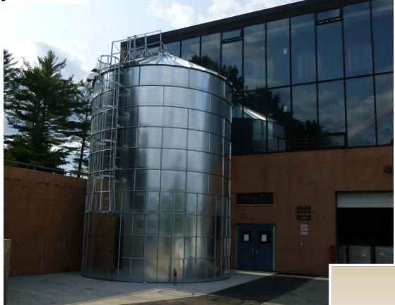
**Exterior Pellet Storage Bin** with Auger Feed to Boiler
