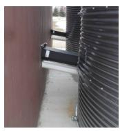
Direct rigid auger feed from bin to boiler
