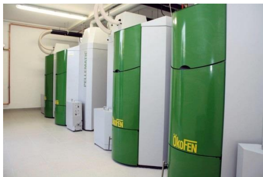
“Staged” or “Cascaded” Pellet Boilers
