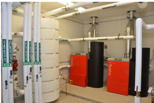
Small Pellet Boilers with Buffer Tank
