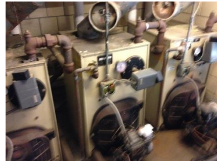
Elementary School Staged Oil Boilers
