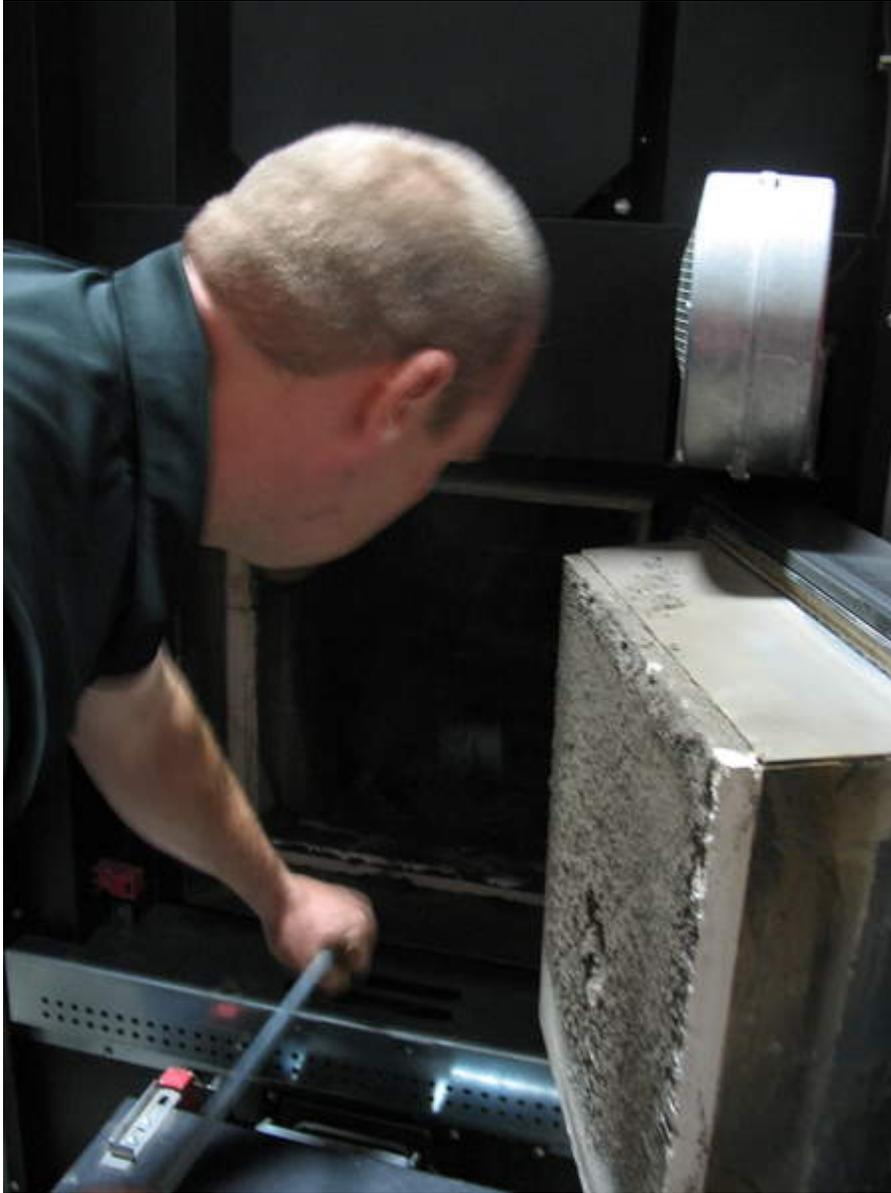
*Photo by: Kerry Miller* Toby Wells, an employee of Froling Energy, demonstrates how to clean a wood burning/hot water boiler at Charlestown's Whelen Engineering. Once a week, he said, ash needs to be scraped out of the boilers. Froling installed the boilers at the company, which heat three quarters of its 250,000 square-foot campus. The New Hampshire Wood Energy Council hosted a tour Wednesday of places in the area, including Whelen, that operate wood heating systems.
