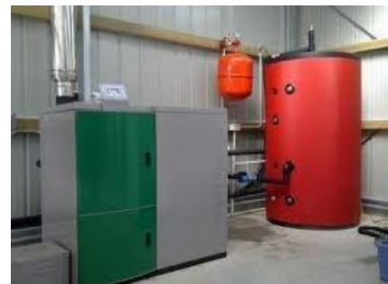
Pellet boiler (green) with buffer tank (red) for hot water storage
