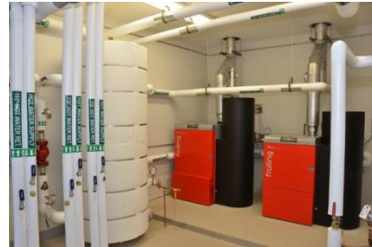
Two pellet boilers (red) with thermal storage (buffer tank, white)
