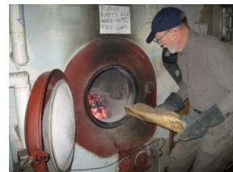
Loading a GARN boiler (not at Sanborn Mills Farm)
